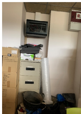
Armari rack de PB
